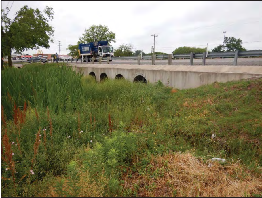
Photograph 17: View looking west toward Crossing 5 - tributary to Pecan Creek (US 377 southbound side).
