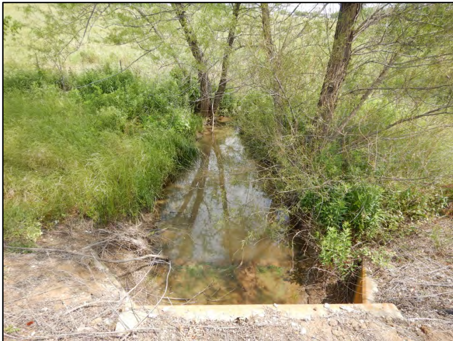
Photograph 90: View looking east along US 377 east ROW near STA. 768+00. The TESCP/EMST Mapper classifies portions of the unmaintained and woody vegetation, and water as Crosstimbers Woodland and Forest. The water and woody and unmaintained vegetation within the depression better fits the Riparian classification. The unmaintained vegetation away from the channel better fits the Disturbed Prairie classification. Date of photograph: 5/13/2020
