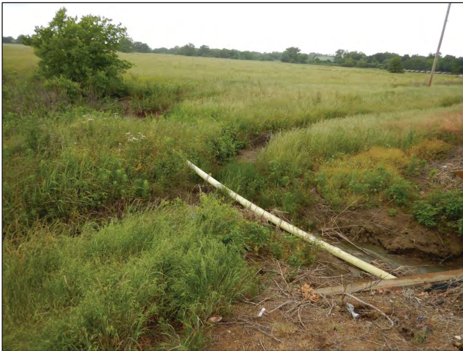
Photograph 54: View looking west toward Crossing 16 – tributary to Cantrell Slough (US 377 southbound side).
