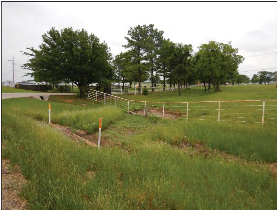
Photograph 34: View looking northeast toward Crossing 10 - tributary to Pecan Creek (US 377 northbound side).
