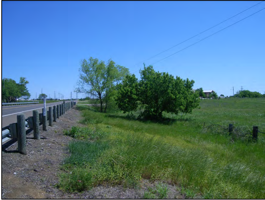
Photograph 91: View looking north along US 377 east ROW near STA. 769+00. The TESCP/EMST Mapper classifies portions of the roadway, and woody, maintained and unmaintained vegetation as Crosstimbers Woodland and Forest. The roadway and typically maintained vegetation within the right-of-way better fit the Urban classification. The woody and unmaintained vegetation better fits the Disturbed Prairie classification. Date of photograph: 4/29/2020
