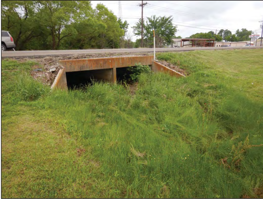
Photograph 39: View looking northwest toward Crossing 12A - tributary to Pecan Creek (US 377 northbound side).
