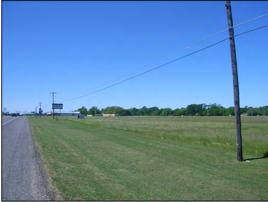
Photograph 11: View looking south along US 377 west ROW from STA. 166+00. The TЕСP/EMST Mapper classifies portions of the roadway and maintained vegetation as Crosstimbers Woodland and Forest. The roadway and vegetation better fit the Urban classification. Date of photograph: 4/29/2020
