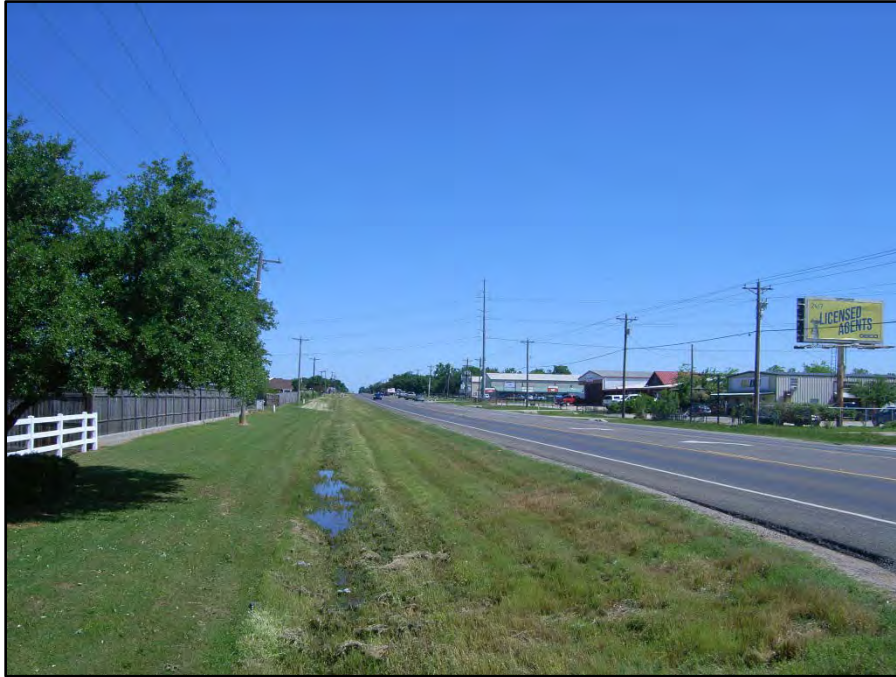
Photograph 71: View looking north along US 377 west ROW near STA. 667+00. The TESCP/EMST Mapper classifies portions of the roadway, and maintained vegetation as Crosstimbers Woodland and Forest. The roadway and maintained vegetation better fit the Urban classification. Date of photograph: 4/29/2020
