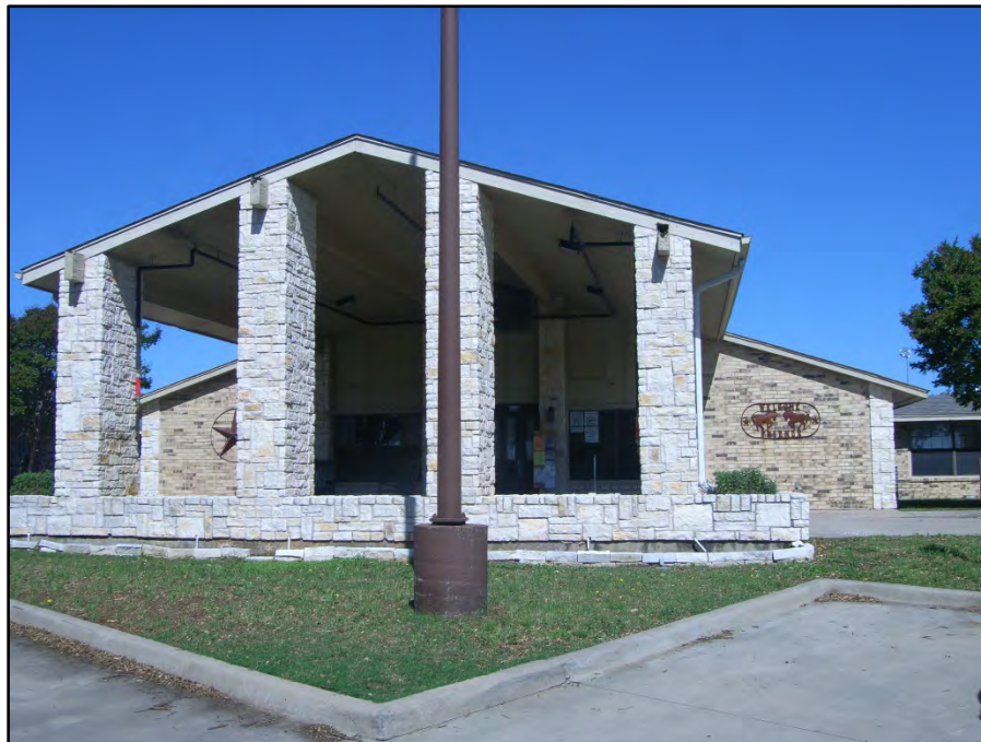
Photograph 1: View looking northwest from a parking lot off Business 377 towards Countryside Nursing & Rehabilitation (ID 3) at 1700 N Washington St, Pilot Point, TX 76258. Date of photograph: 4/29/20.
