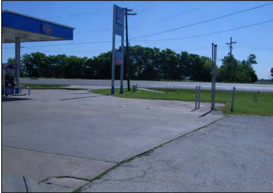
Photograph 7: View looking northeast towards the tank hold of the Evan's Stop N Go LPST and PST site at 110 N. US 377, Pilot Point, TX 76258 (Map ID 20). Date of photograph: 4/29/20.
