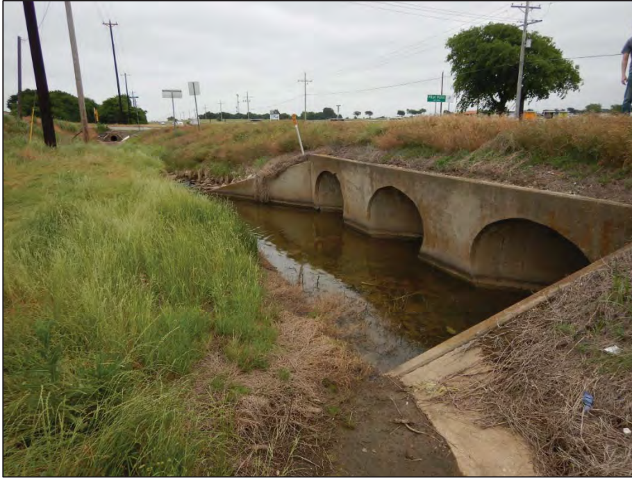
Photograph 25: View looking east toward Crossing 8 - tributary to Pecan Creek (US 377 southbound side).
