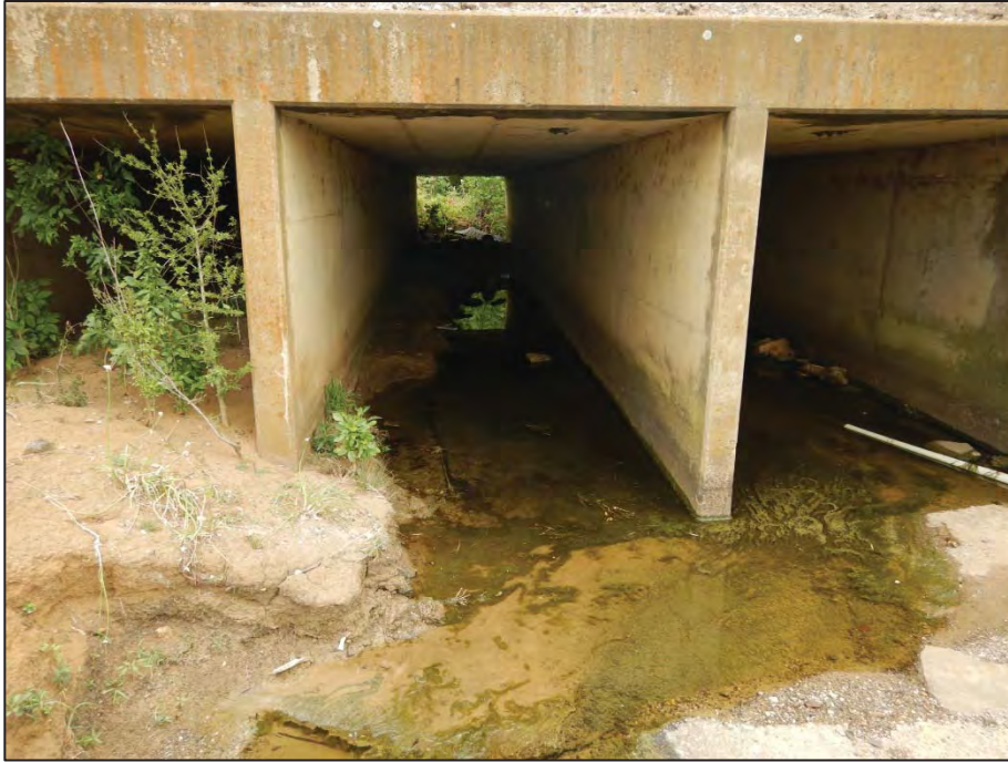
Photograph 43: View looking east toward Crossing 13 - Running Branch (US 377 southbound side).
