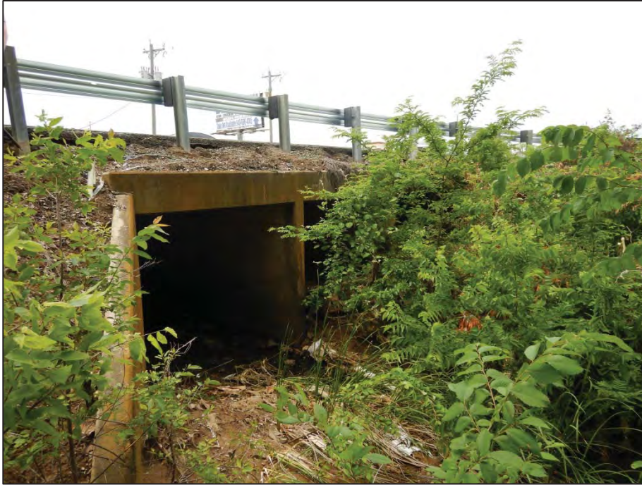
Photograph 45: View looking west toward Crossing 13 – Running Branch (US 377 northbound side).
