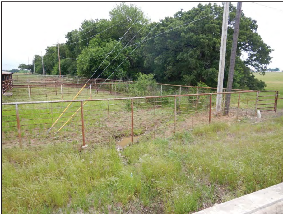
Photograph 22: View looking southeast toward Crossing 6 – tributary to Pecan Creek (US 377 southbound side).
