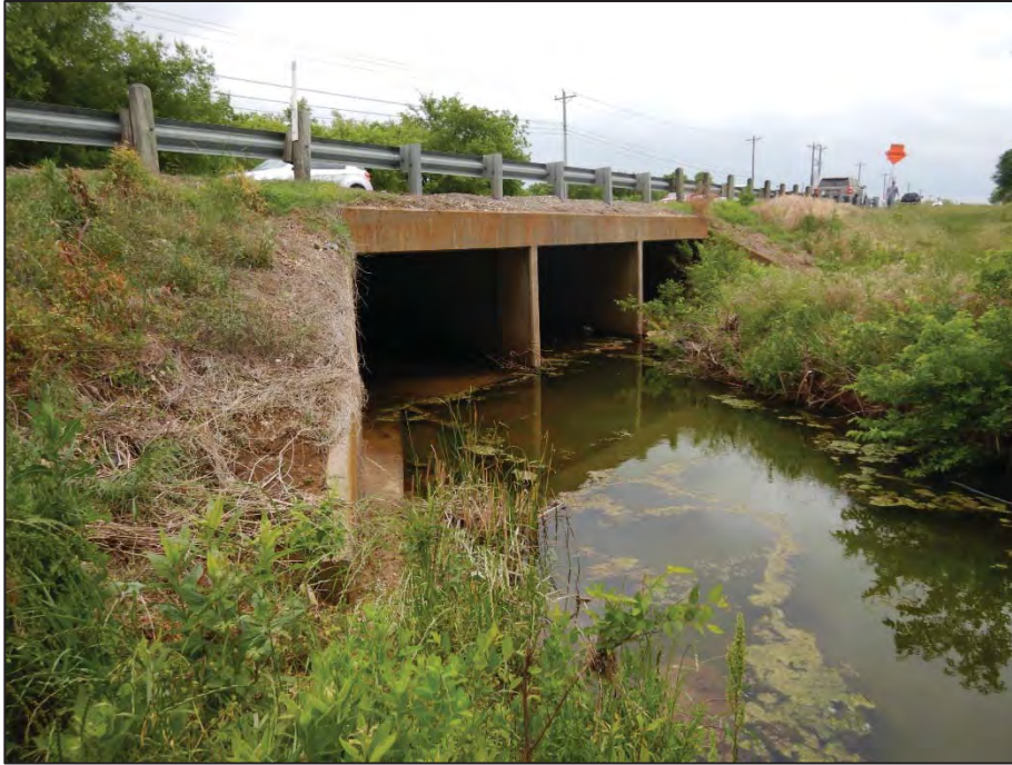
Photograph 47: View looking southeast toward Crossing 14 - tributary to Pecan Creek (US 377 southbound side).
