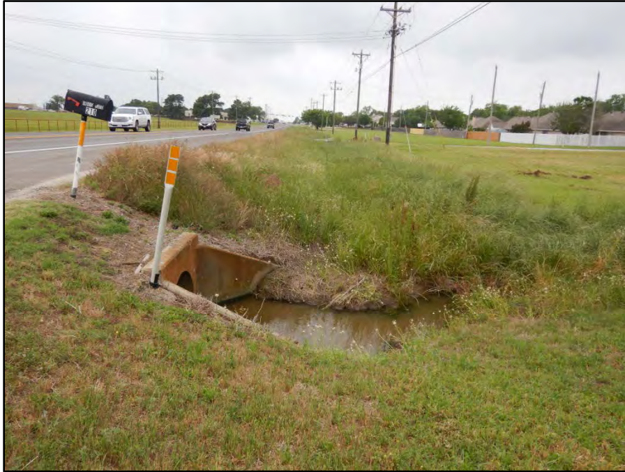
Photograph 57: View looking southwest along US 377 west ROW near STA. 545+00. The TЕСP/EMST Mapper classifies the unmaintained vegetation and water as Urban. The unmaintained vegetation and water better fit the Riparian classification. Date of photograph: 5/13/2020
