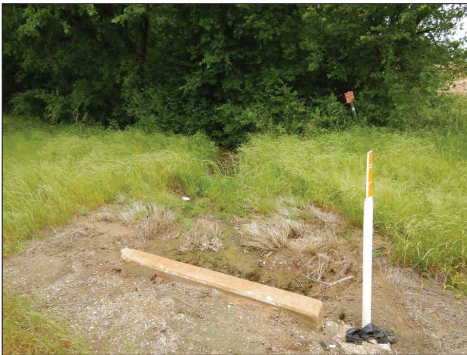
Photograph 24: View looking northeast toward Crossing 7 - tributary to Pecan Creek (US 377 northbound side).
