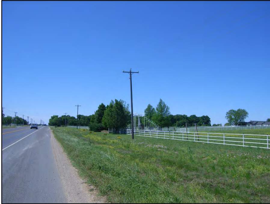
Photograph 79: View looking south along US 377 west ROW near STA. 702+50. The TESCP/EMST Mapper classifies portions of the roadway and maintained vegetation as Crosstimbers Woodland and Forest. The roadway and vegetation better fit the Urban classification. Date of photograph: 4/29/2020
