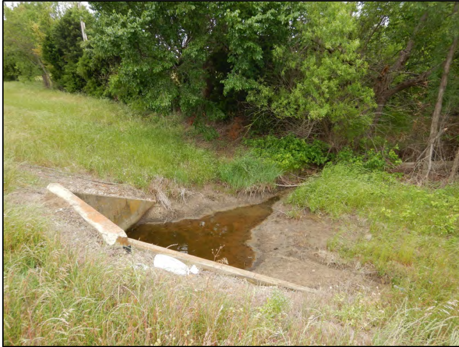
Photograph 55: View looking west along US 377 west ROW near STA. 513+50. The TESCP/EMST Mapper classifies portions of the woody vegetation and water as Urban and Crosstimbers Woodland and Forest. The woody vegetation surrounding the channel better fits the Riparian classification. The woody vegetation beyond the channel fits the Crosstimbers Woodland and Forest classification. Date of photograph: 5/13/2020
