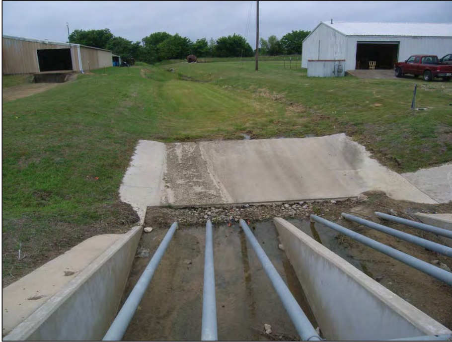
Photograph 5: View looking west toward Crossing 2 - tributary to Pecan Creek (US 377 southbound side).
