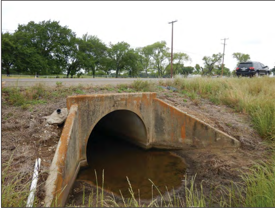
Photograph 35: View looking southeast toward Crossing 11 – tributary to Pecan Creek (US 377 southbound side).
