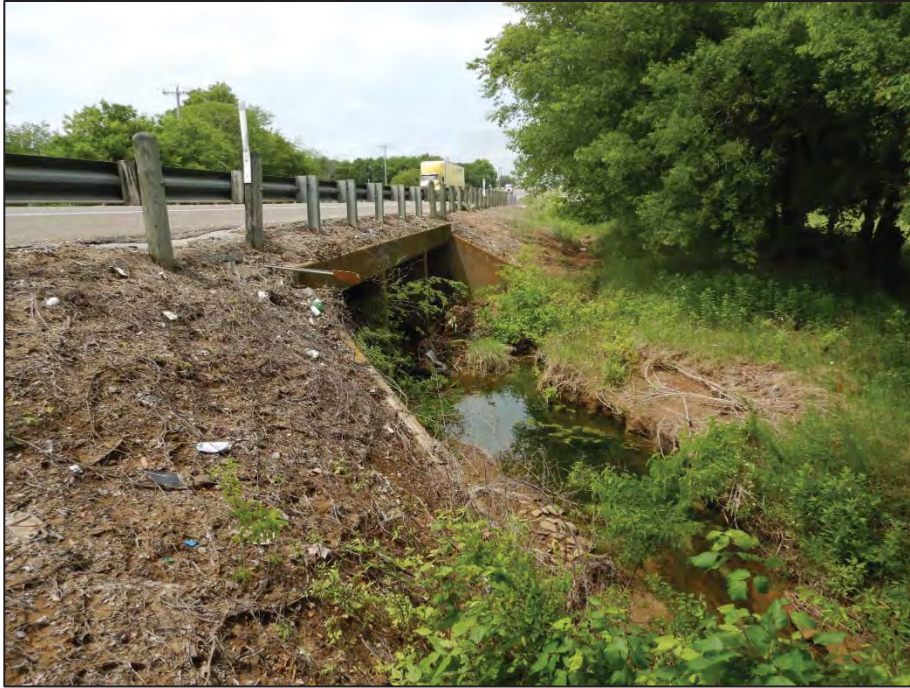
Photograph 49: View looking northwest toward Crossing 14 - tributary to Pecan Creek (US 377 northbound side).
