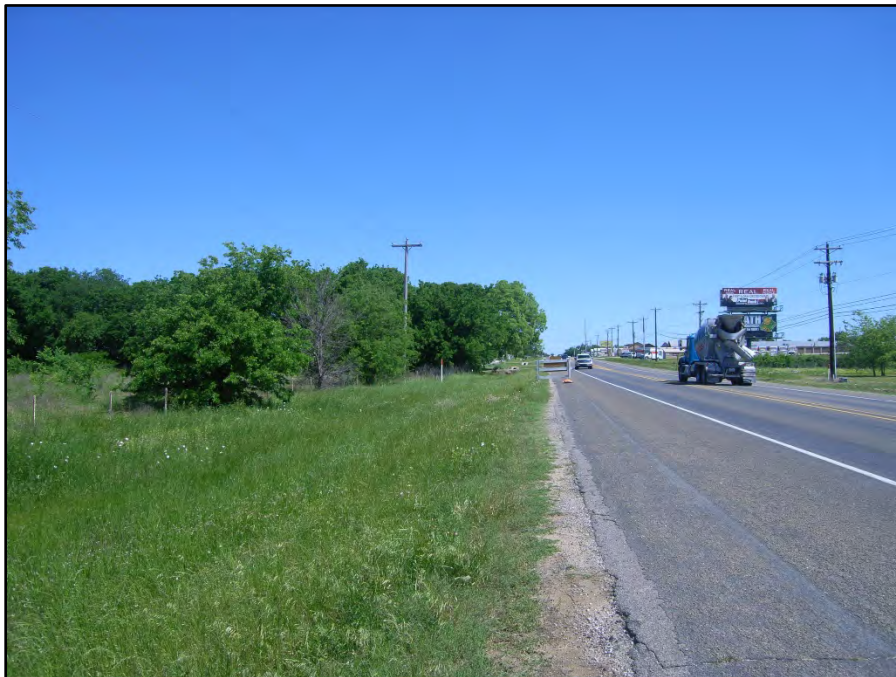
Photograph 72: View looking north along US 377 west ROW near STA. 680+00. The TESCP/EMST Mapper classifies portions of the roadway, maintained and woody vegetation as Crosstimbers Woodland and Forest. The woody vegetation fits the Crosstimbers Woodland and Forest classification. The roadway and maintained vegetation better fit the Urban classification. Date of photograph: 4/29/2020
