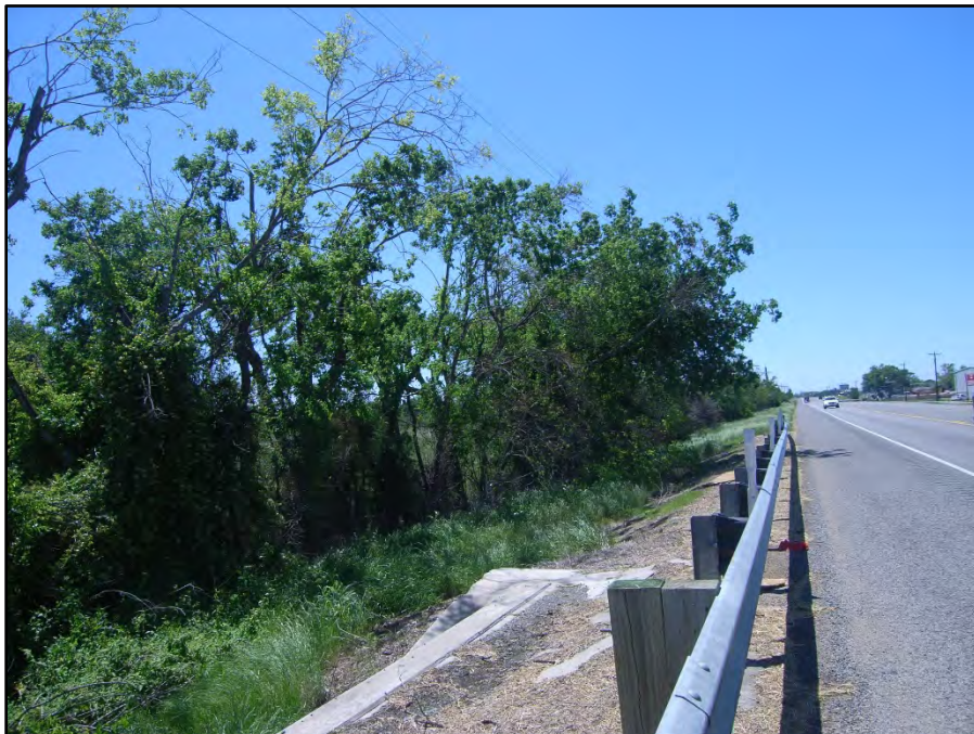
Photograph 8: View looking southeast from the US 377 east ROW near STA. 148+00. The TESCP/EMST Mapper classifies the roadway and unmaintained and woody vegetation as Urban; however, the unmaintained vegetation within the ditch better fits the Riparian classification. The woody vegetation better fits the Disturbed Prairie classification. Date of photograph: 4/29/2020
