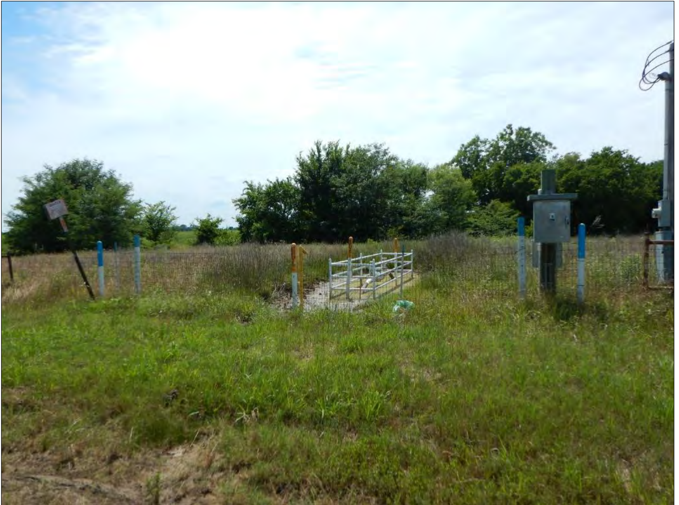
18. Gas line and utilities along the ROW (facing west).
