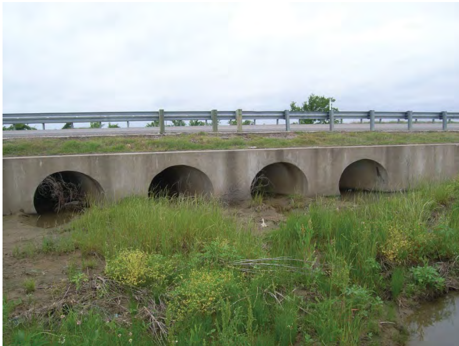
Photograph 2: View looking west toward Crossing 1 - tributary to Pecan Creek (US 377 northbound side).
