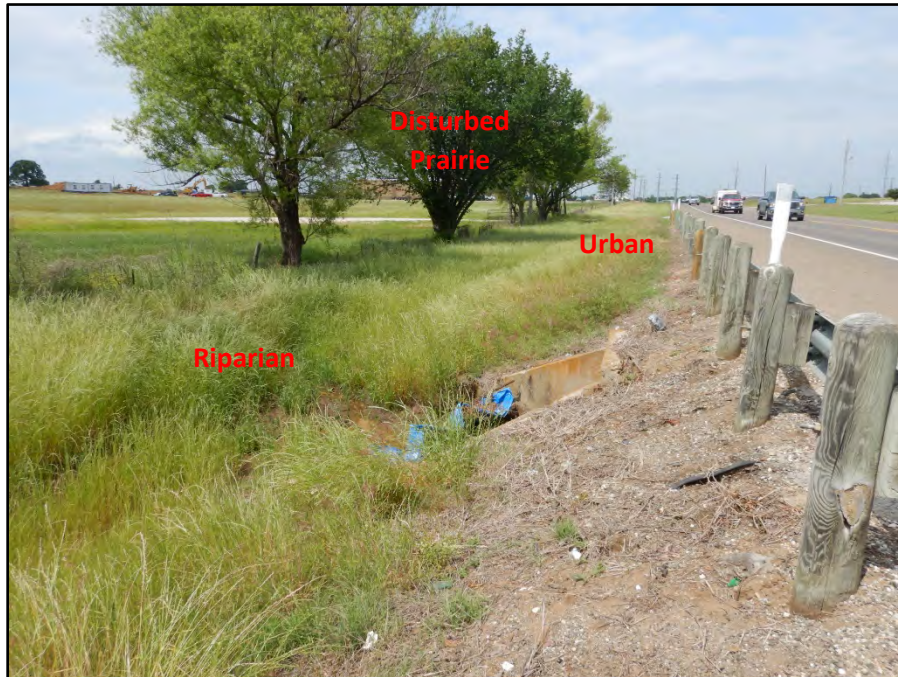
Photograph 89: View looking north along US 377 west ROW near STA. 769+00. The TESCP/EMST Mapper classifies portions of the roadway, and maintained, unmaintained and woody vegetation as Crosstimbers Woodland and Forest. The roadway and typically maintained vegetation better fit the Urban classification. The woody vegetation better fits the Disturbed Prairie classification. The unmaintained vegetation in the depression better fits the Riparian classification. Date of photograph: 5/13/2020
