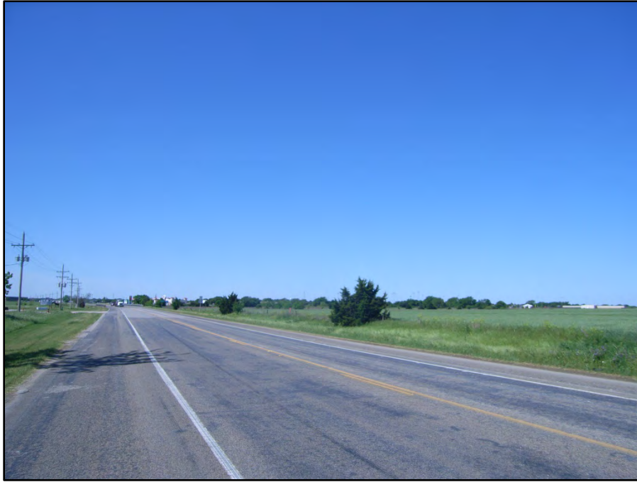
Photograph 1: View looking south along the US 377 east ROW from near STA. 96+00. The TESCP/EMST Mapper classifies the roadway and vegetation as Disturbed Prairie and Tallgrass Prairie, Grassland; however, the roadway better fits the Urban classification. The unmaintained vegetation fits the Disturbed Prairie classification. Date of photograph: 4/29/2020
