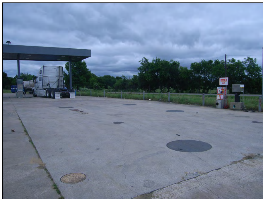
Photograph 16: View looking northeast towards the tank hold of a Circle K (formerly US 380 Travel Center CK 119), a PST site at 6500 US Highway 380, Cross Roads, TX 76227 (Map ID 31). Date of photograph: 5/26/20.
