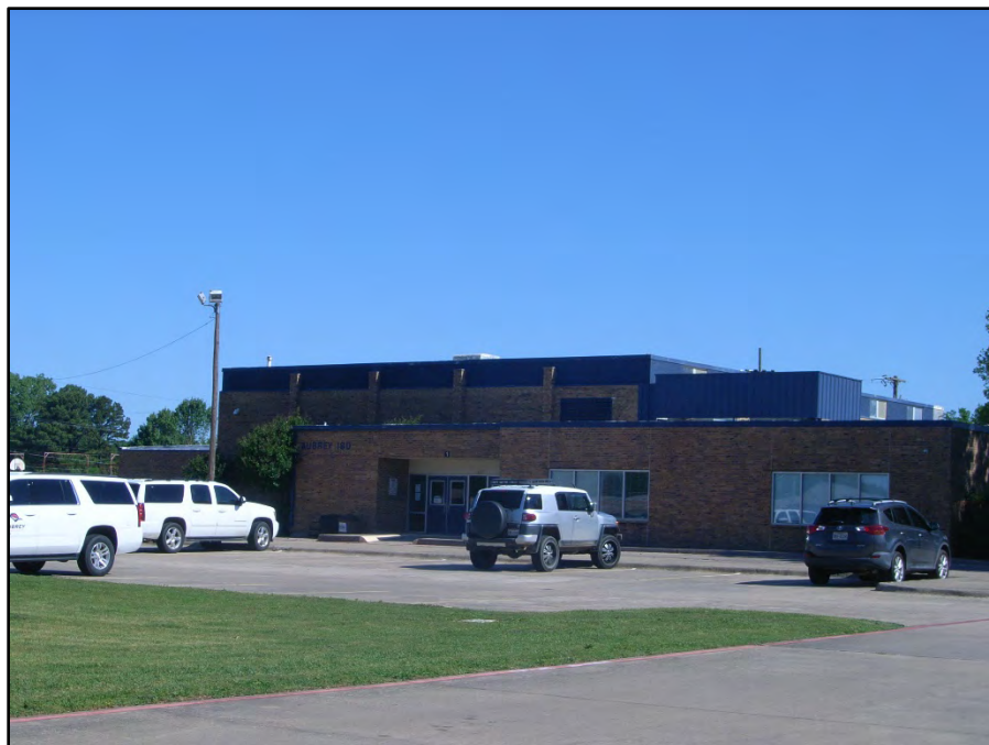
Photograph 8: View looking west from a parking lot off US 377 towards the Early Bird Learning Center (ID 41) at 415 Tisdell Ln, Aubrey, TX 76227. Date of photograph: 4/29/20.
