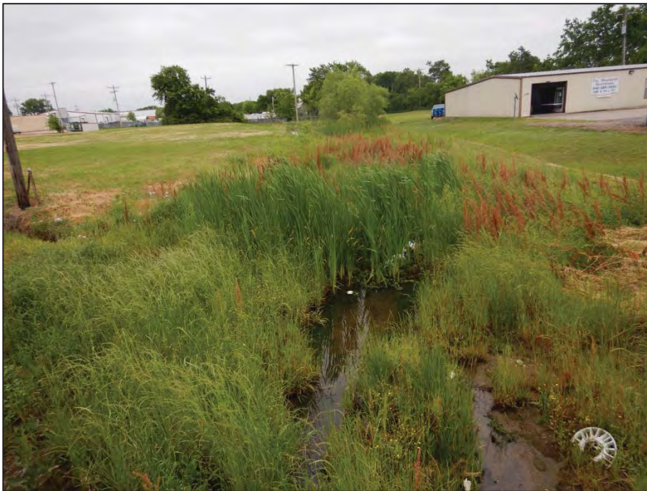
Photograph 18: View looking southeast toward Crossing 5 - tributary to Pecan Creek (US 377 southbound side).
