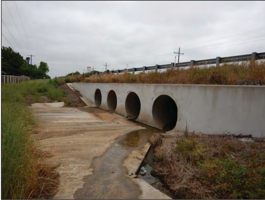
Photograph 15: View looking northeast toward Crossing 5 - tributary to Pecan Creek (US 377 southbound side).
