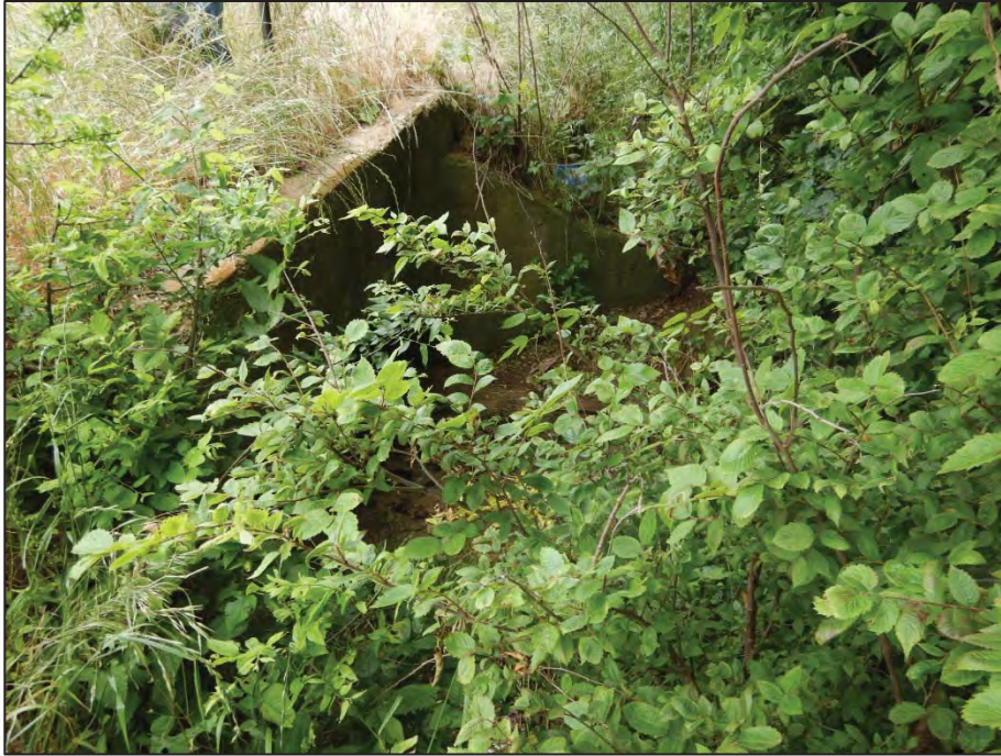
Photograph 19: View looking east toward Crossing 6 – tributary to Pecan Creek (US 377 northbound side).
