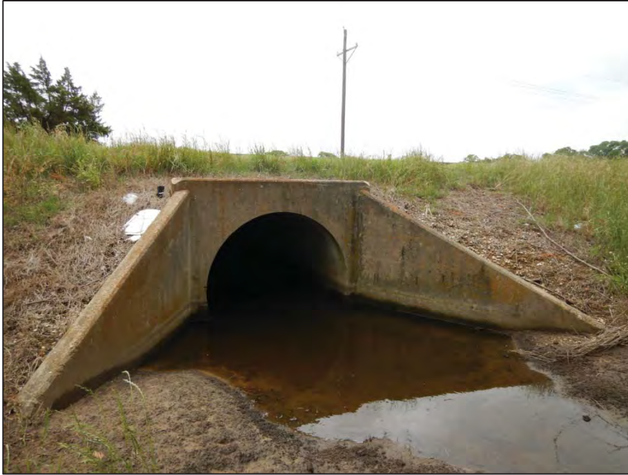
Photograph 37: View looking northwest toward Crossing 11 – tributary to Pecan Creek (US 377 northbound side).
