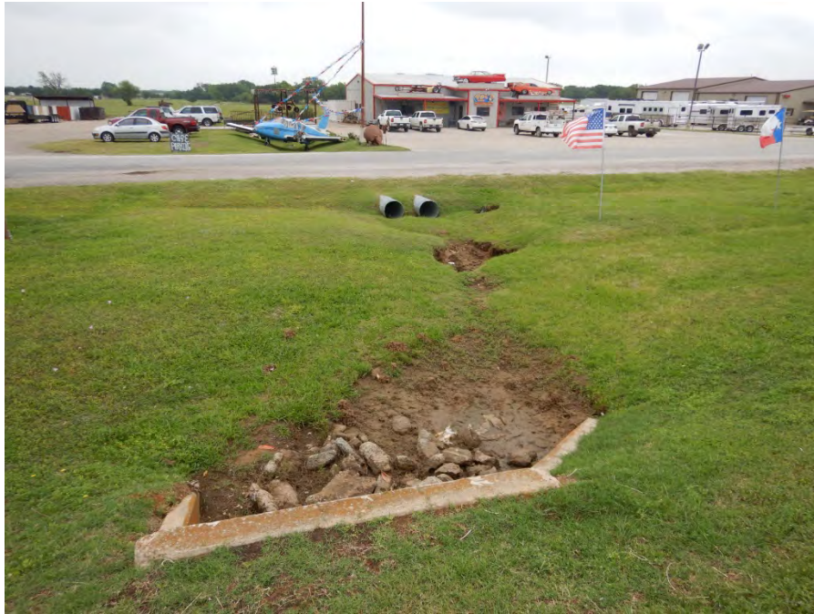
Photograph 45: View looking northeast along US 377 east ROW near STA. 455+50. The TESCP/EMST Mapper classifies portions of the maintained vegetation as Riparian and Crosstimbers Woodland and Forest. The maintained vegetation better fits the Urban classification. Date of photograph: 5/13/2020
