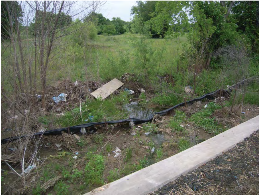
Photograph 3: View looking east toward Crossing 2 - tributary to Pecan Creek (US 377 northbound side).
