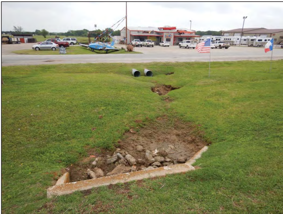
Photograph 30: View looking southeast toward Crossing 9 – tributary to Pecan Creek (US 377 southbound side).
