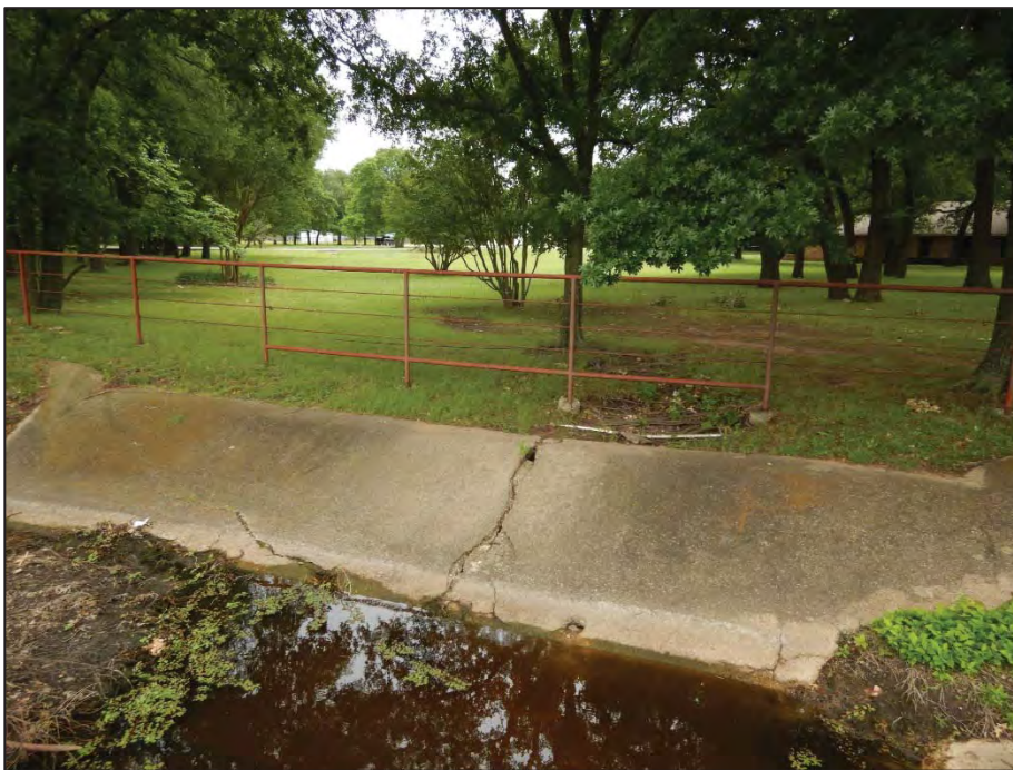
Photograph 32: View looking southwest toward Crossing 10 - tributary to Pecan Creek (US 377 southbound side).
