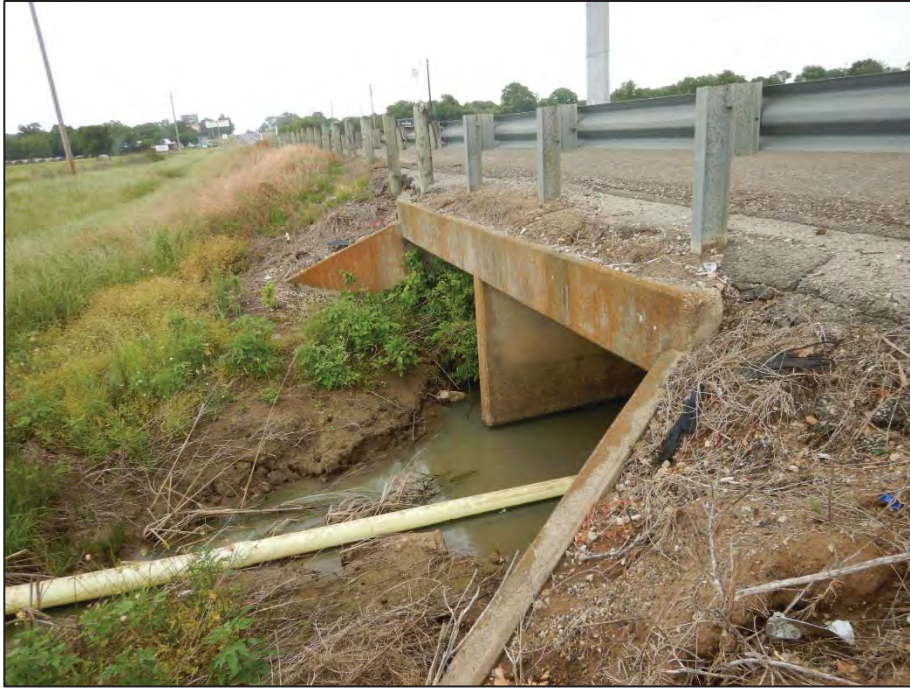
Photograph 53: View looking north toward Crossing 16 – tributary to Cantrell Slough (US 377 southbound side).
