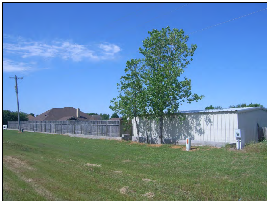
Photograph 28: View looking southwest from US 377 toward a metal shed, and two other storage buildings, potential displacements (Disp. 11) at 855 Sherry Ln S, Krugerville, TX 76227. Date of photograph: 5/6/20
