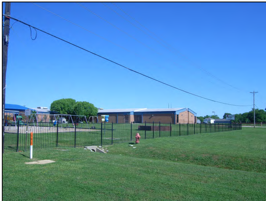
Photograph 11: View looking north from a parking lot off US 377 towards HL Brockett Elementary School (ID 55) at 900 Chestnut St, Aubrey, TX 76227. Date of photograph: 4/29/20.
