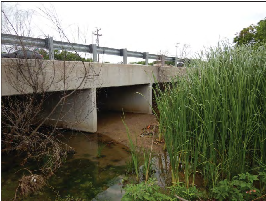
Photograph 10: View looking northwest toward Crossing 3 - tributary to Pecan Creek (US 377 northbound side).
