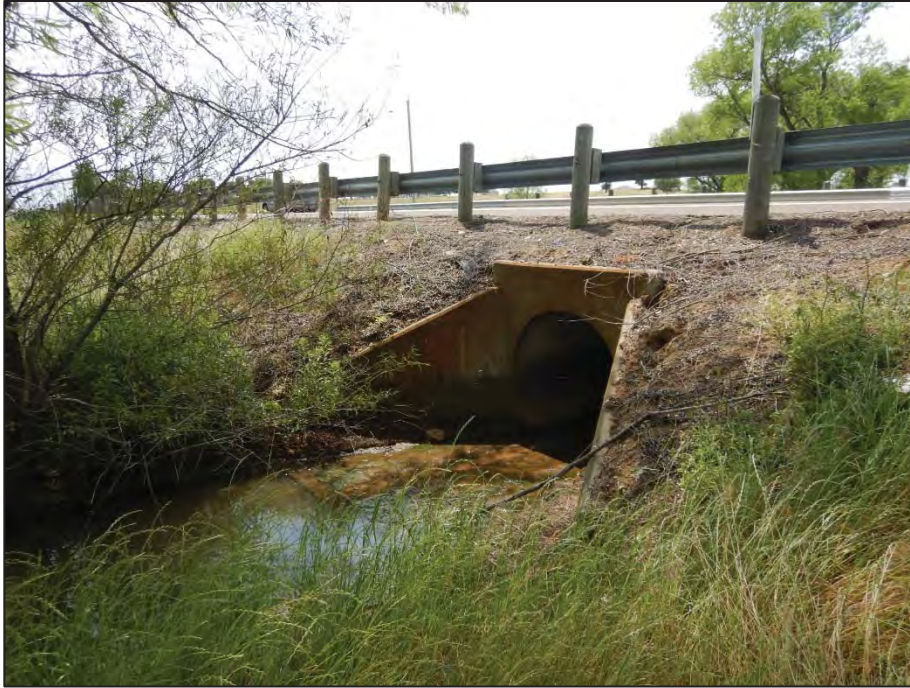
Photograph 57: View looking northwest toward Crossing 17 - tributary to Cantrell Slough (US 377 northbound side).
