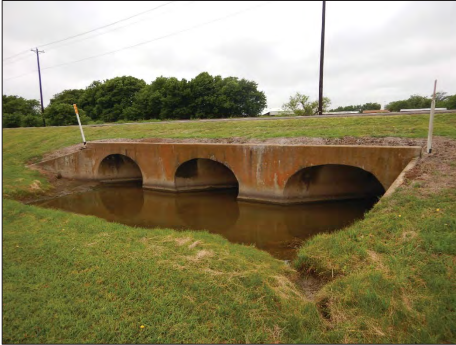
Photograph 27: View looking west toward Crossing 8 - tributary to Pecan Creek (US 377 northbound side).
