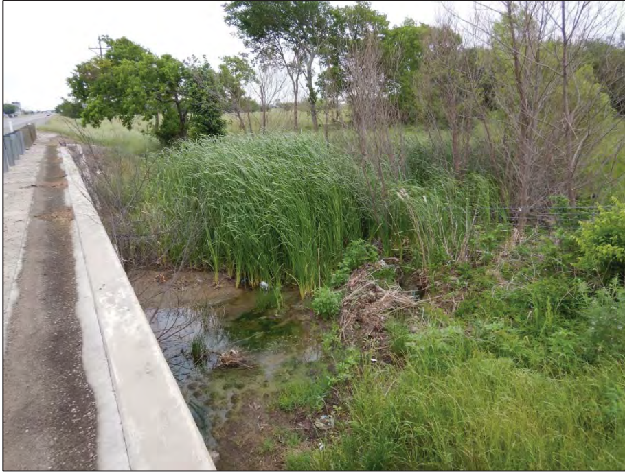
Photograph 9: View looking north toward Crossing 3 - tributary to Pecan Creek (US 377 northbound side).
