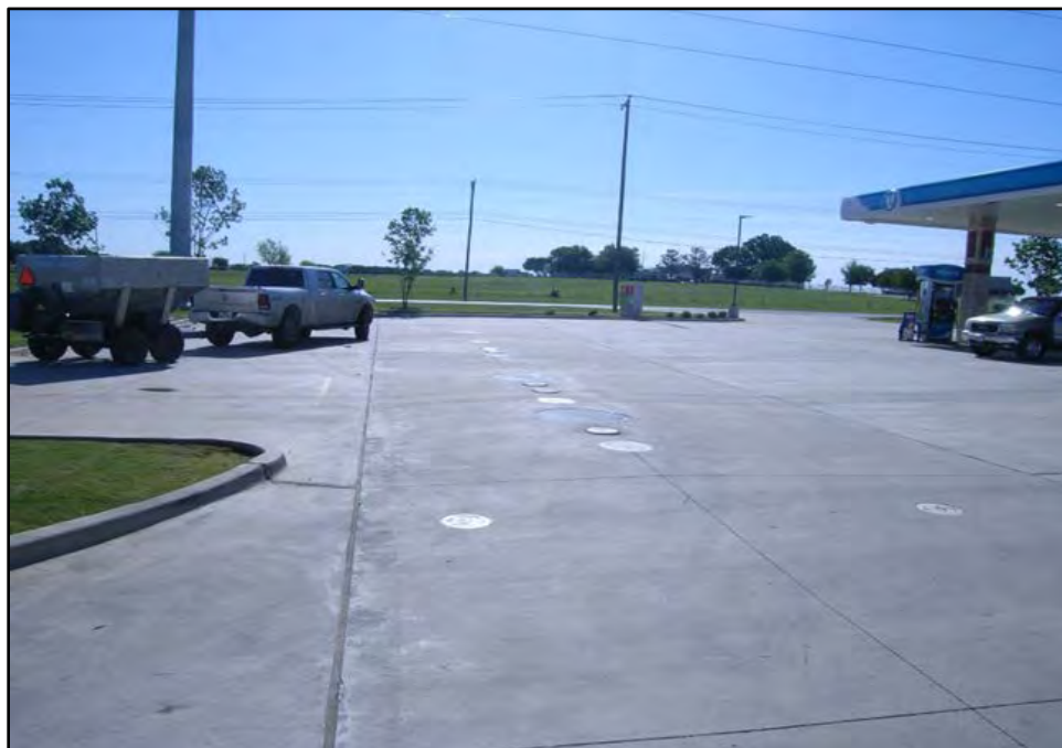
Photograph 14: View looking east towards the tank hold of the Circle K Store 2741876 PST site at 7500 S. US 377, Aubrey, TX 76227 (Map ID 29). Date of photograph: 4/29/20.
