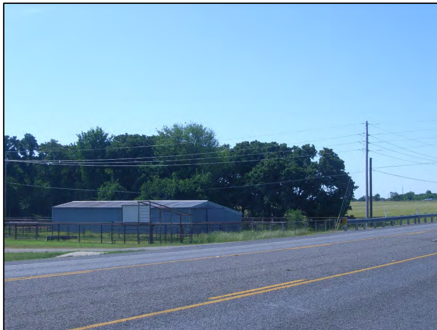
Photograph 21: View looking southeast from US 377 toward a metal barn that is a potential displacement (Disp. 3) at 1311 S US 377, Pilot Point, TX 76258. Date of photograph: 5/6/20
