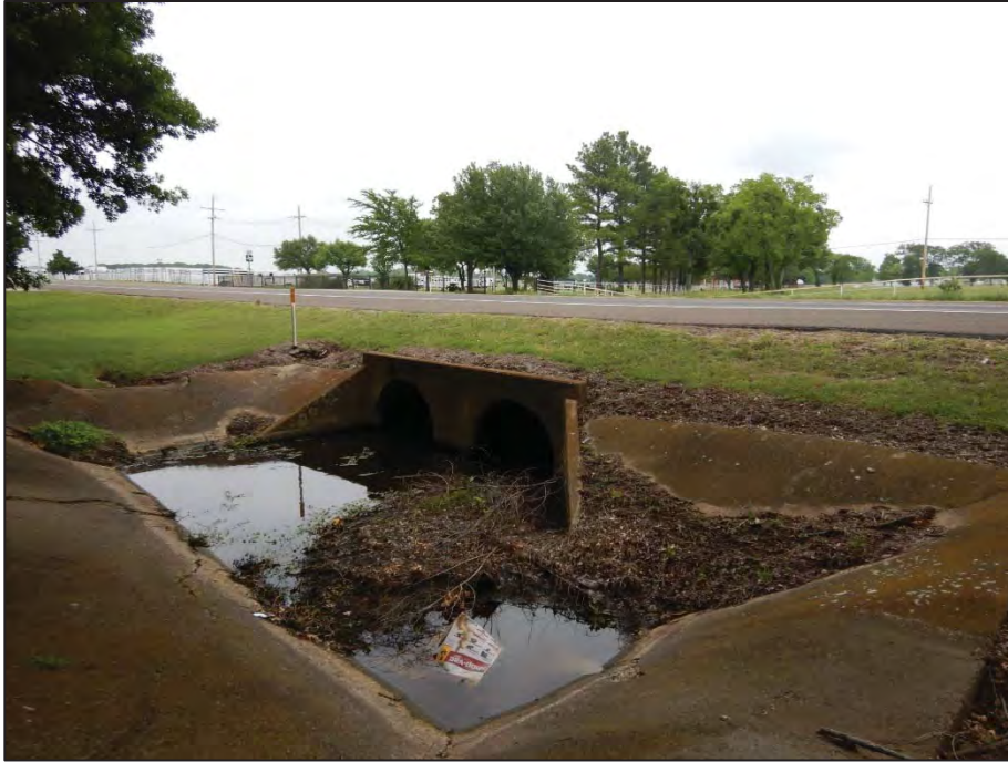
Photograph 31: View looking northeast toward Crossing 10 - tributary to Pecan Creek (US 377 southbound side).
