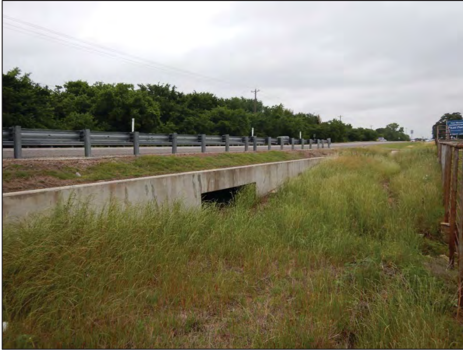
Photograph 21: View looking northwest toward Crossing 6 – tributary to Pecan Creek (US 377 southbound side).
