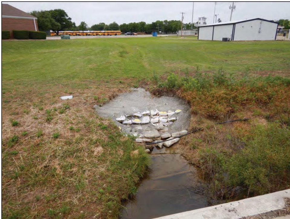
Photograph 12: View looking northwest toward Crossing 4 - tributary to Pecan Creek (US 377 southbound side).
