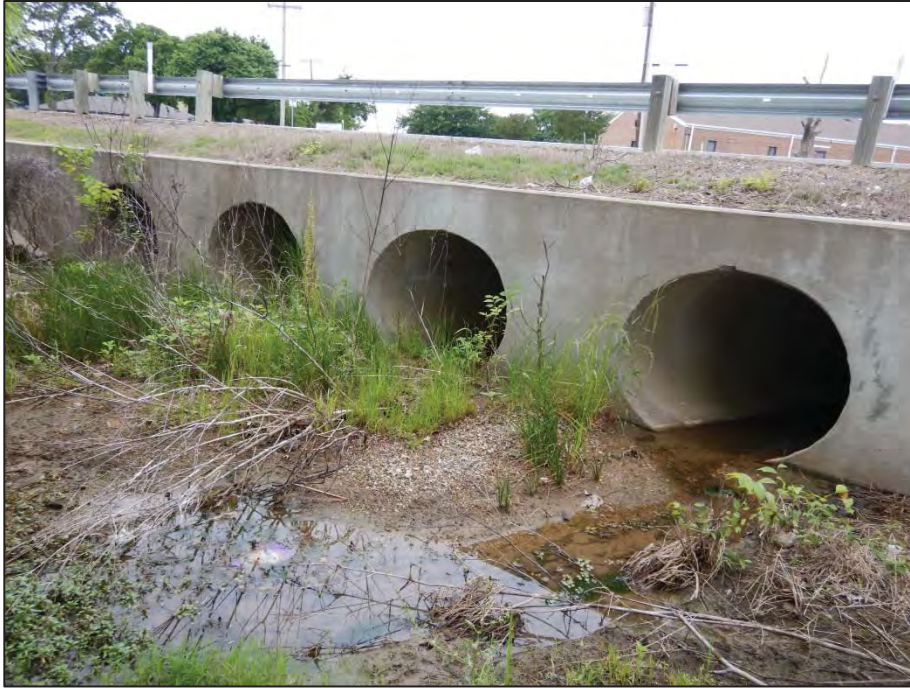
Photograph 13: View looking north toward Crossing 4 - tributary to Pecan Creek (US 377 northbound side).
