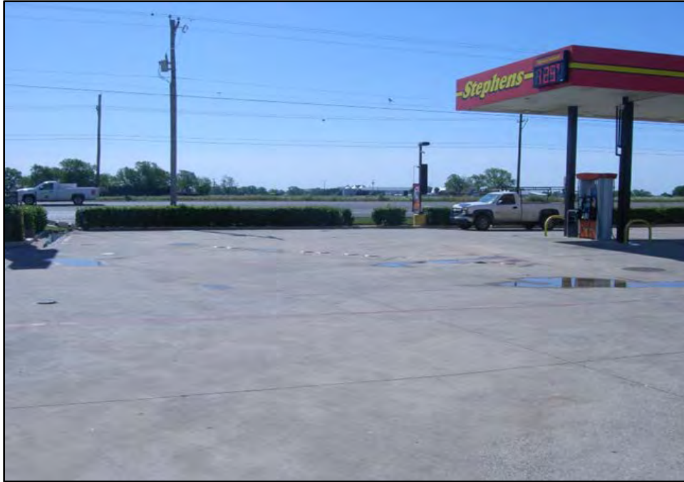
Photograph 9: View looking southeast towards the tank hold of the Stephen's Fuel Center LPST and PST site at 442 S. US 377, Pilot Point, TX 76258 (Map ID 26). Date of photograph: 4/29/20.
