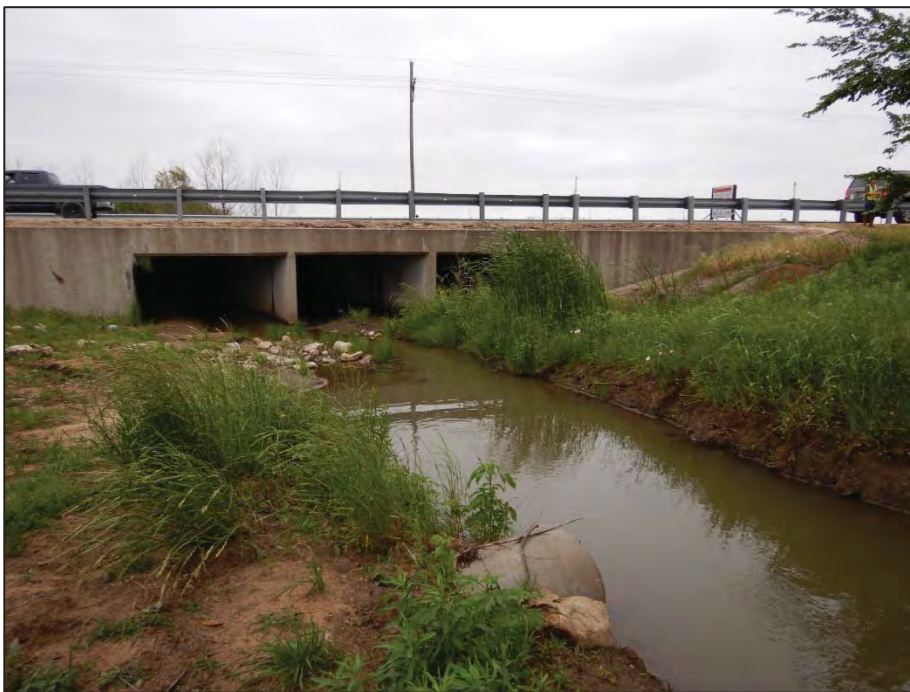
Photograph 8: View looking east toward Crossing 3 - tributary to Pecan Creek (US 377 southbound side).
