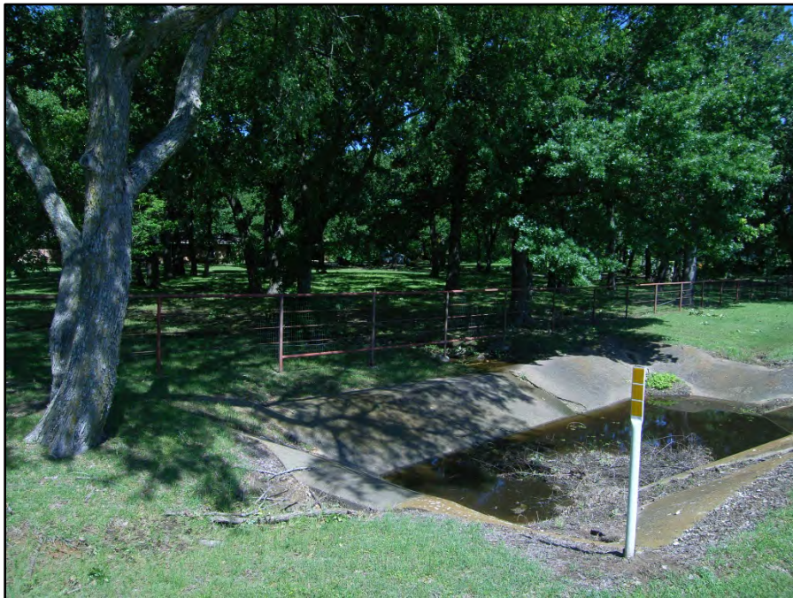
Photograph 48: View looking north along US 377 west ROW near STA. 471+00. The TESCP/EMST Mapper classifies portions of the maintained and woody vegetation, and water as Riparian and Crosstimbers Woodland and Forest. The woody vegetation fits the Crosstimbers Woodland and Forest classification. The maintained vegetation and water better fit the Urban classification. Date of photograph: 4/29/2020
