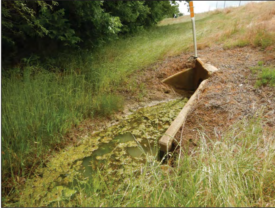
Photograph 59: View looking north toward Crossing 18 – tributary to Cantrell Slough (US 377 northbound side).
