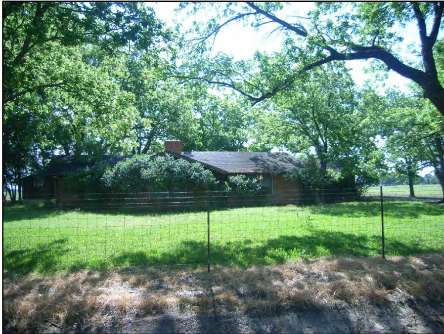
Photograph 29: View looking east from Debbie Ln in Pilot Point toward a home in disrepair, possibly abandoned. Date of photograph: 5/6/20
