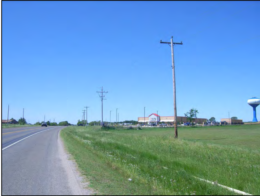
Photograph 87: View looking southwest along US 377 west ROW near STA. 754+00. The TESCP/EMST Mapper classifies portions of the roadway and vegetation as Crosstimbers Woodland and Forest. The roadway and vegetation better fit the Urban classification. Date of photograph: 4/29/2020
