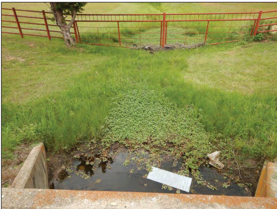
Photograph 38: View looking east toward Crossing 11 – tributary to Pecan Creek (US 377 northbound side).
