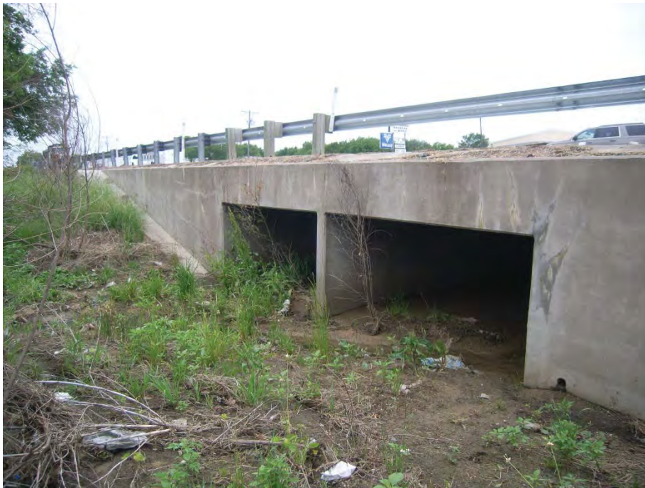
Photograph 4: View looking west toward Crossing 2 - tributary to Pecan Creek (US 377 northbound side).
