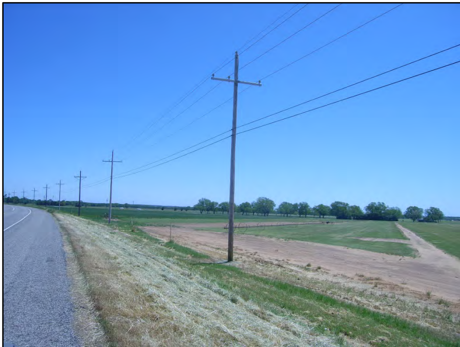
Photograph 14: View looking east along US 377 east ROW near STA. 195+00. The TESCP/EMST Mapper classifies portions of the roadway, and the mowed-maintained and other vegetation as Crosstimbers Woodland and Forest. The roadway and mowed-maintained vegetation better fit the Urban classification. The other vegetation that appears to be a turf farm better fits the Agriculture classification. Date of photograph: 4/29/2020
