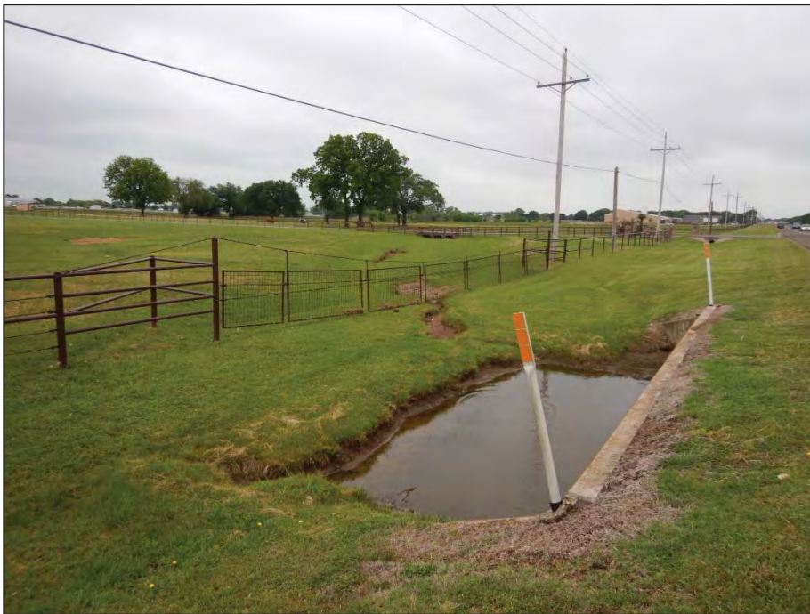
Photograph 28: View looking southeast toward Crossing 8 - tributary to Pecan Creek (US 377 northbound side).
