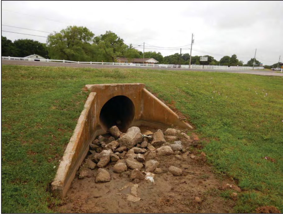
Photograph 29: View looking northwest toward Crossing 9 – tributary to Pecan Creek (US 377 southbound side)
