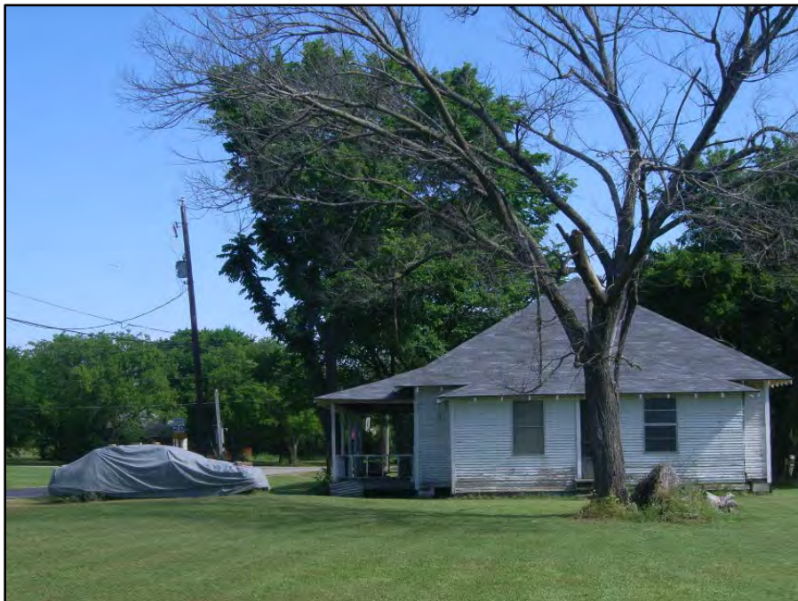
Photograph 30: View looking north from E Walcott St in Pilot Point toward a home in disrepair. Date of photograph: 5/6/20
