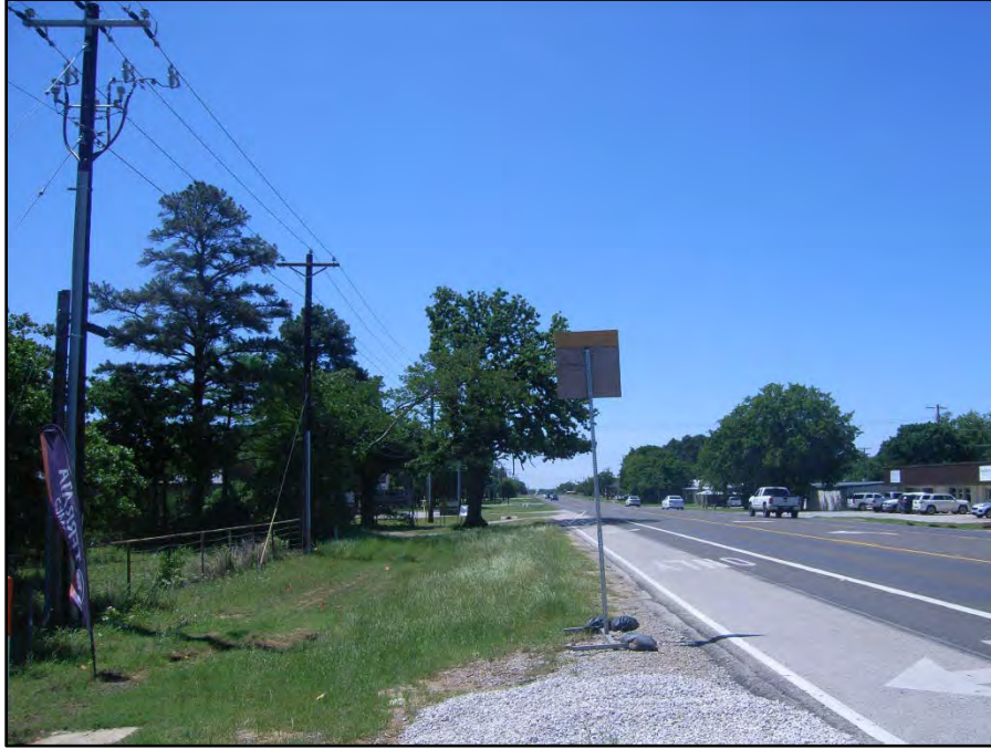
Photograph 67: View looking south along US 377 east ROW near STA. 620+50. The TESCP/EMST Mapper classifies portions of the roadway, and maintained and woody vegetation as Crosstimbers Woodland and Forest. The roadway and maintained vegetation better fit the Urban classification. The woody vegetation fits the Crosstimbers Woodland and Forest classification. Date of photograph: 4/29/2020
