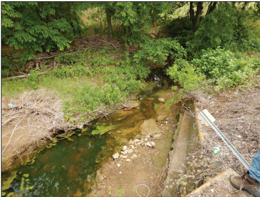
Photograph 50: View looking southeast toward Crossing 14 - tributary to Pecan Creek (US 377 northbound side).
