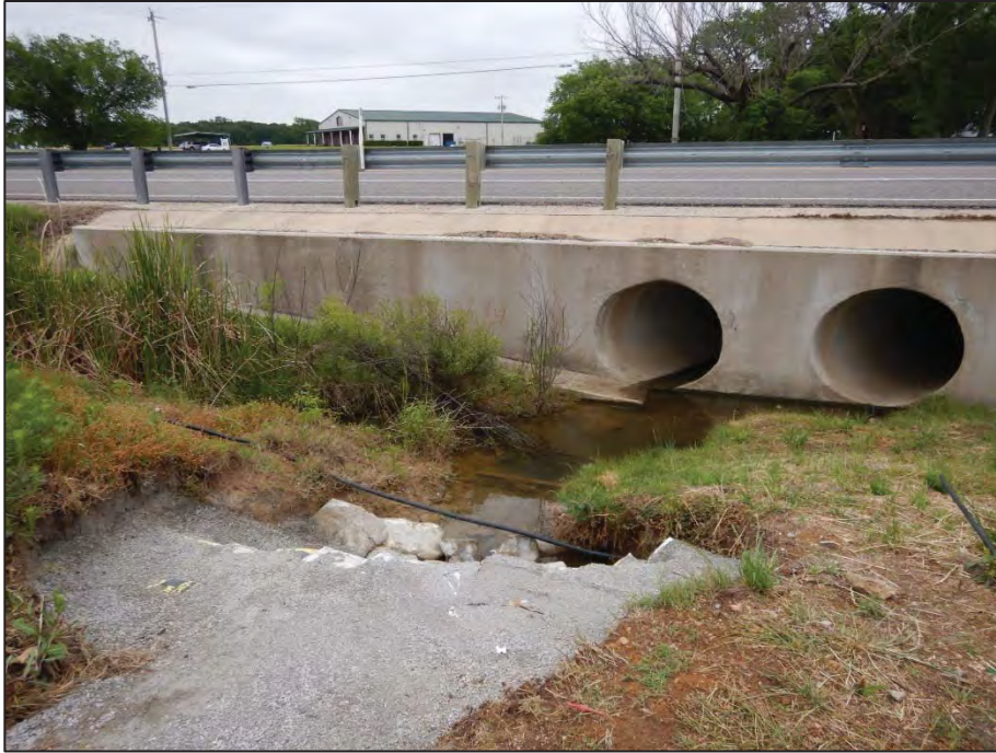
Photograph 11: View looking southeast toward Crossing 4 - tributary to Pecan Creek (US 377 southbound side).
