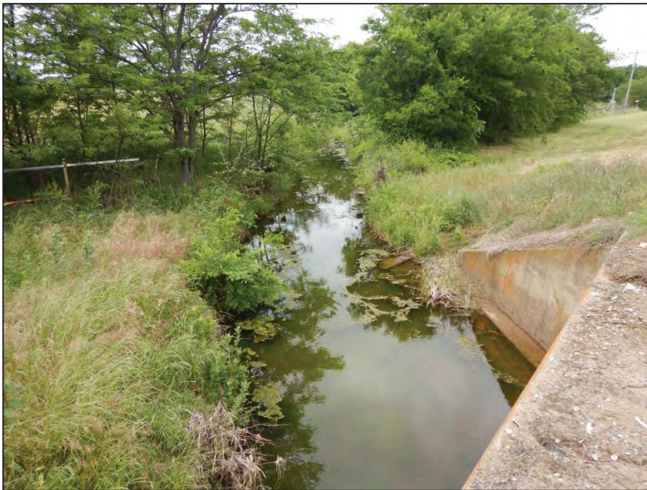
Photograph 48: View looking northwest toward Crossing 14 - tributary to Pecan Creek (US 377 southbound side).
