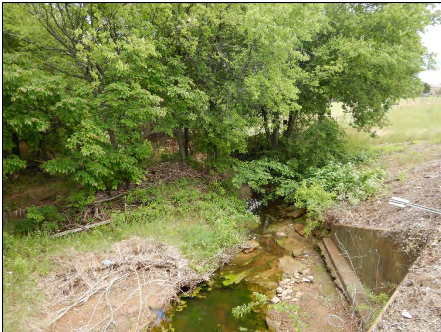
Photograph 76: View looking southeast along US 377 east ROW near STA. 684+00. The TЕСP/EMST Mapper classifies maintained, unmaintained and woody vegetation, and water as Urban and Riparian. The woody vegetation and water near the channel fit the Riparian classification. The woody vegetation away from the channel better fits the Disturbed Prairie classification. The maintained vegetation fits the Urban classification. Date of photograph: 5/13/2020
