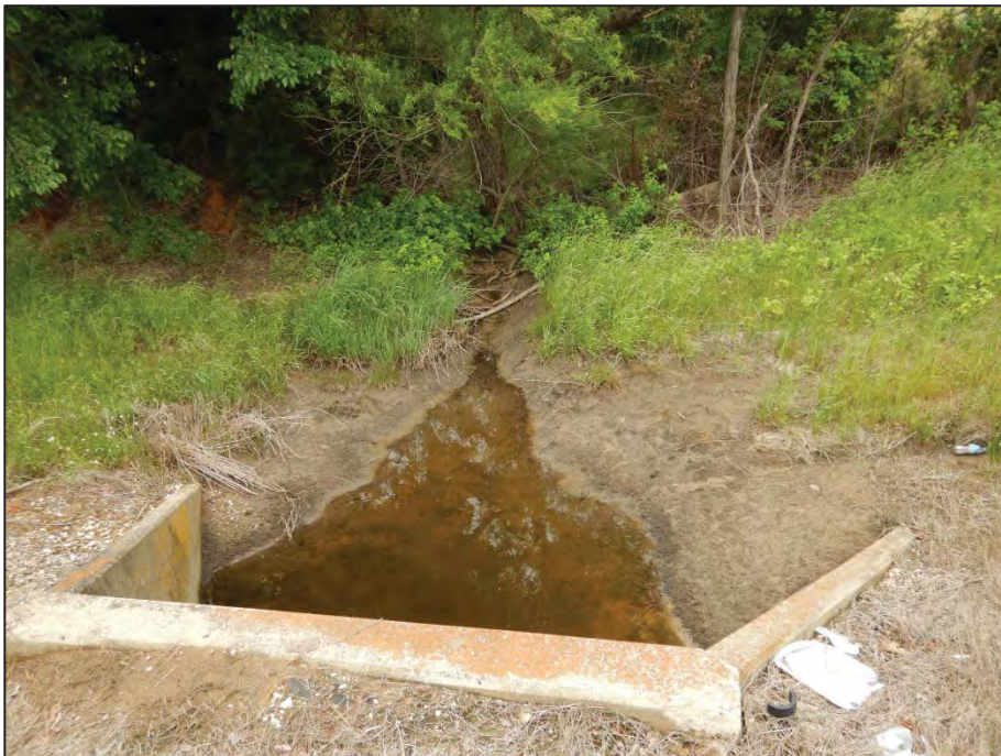
Photograph 36: View looking northwest toward Crossing 11 – tributary to Pecan Creek (US 377 southbound side).
